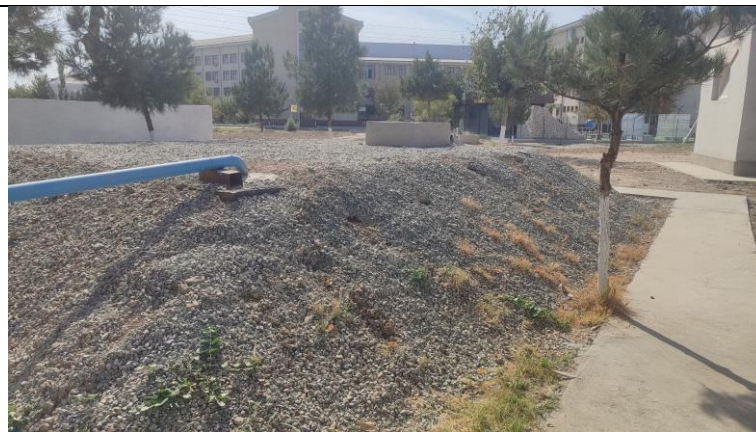
In Ground Water Tank (Karshi State University)
